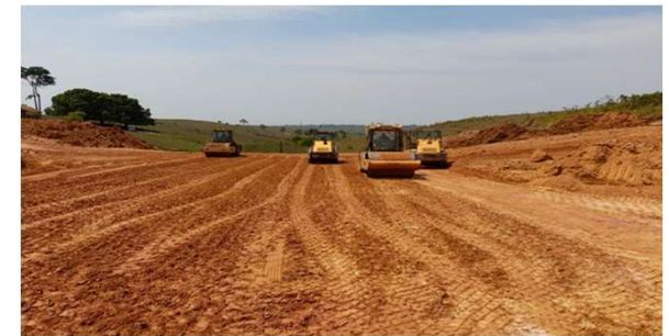
Const. Carretera Porvenir – Puerto Rico; Tramo IB: San Miguel – Puerto Rico
